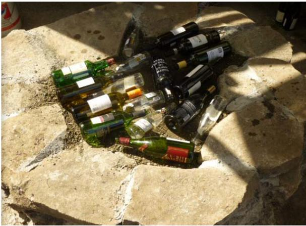
Once the base was built we laid bottles inside the opening and stuffed a mixture of clay, sawdust and water in between the bottles. We then covered this layer with sand and leveled it. This acts as an insulation layer to keep the base from soaking up the heat of the oven.
